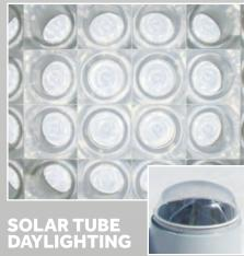
Solar tube skylights pull a dramatic amount of "ducted daylight" into the second floor open office space producing up to 20,500 lumens each. In this regularly occupied space, the solar tubes minimize the need for artificial lighting during normal daytime occupancy.
