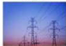
AC Line Power
