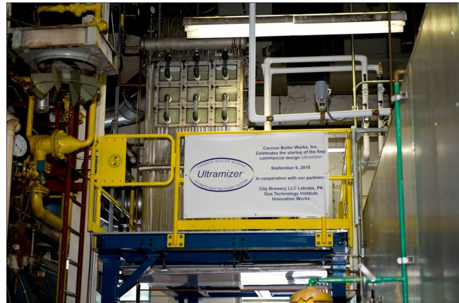
Industrial boiler heat recovery with Ultramizer product at brewery
