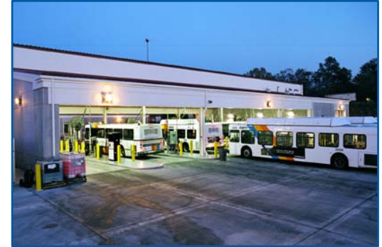
NGV Fuelling Station
